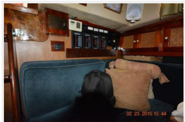
Electric panel aft salon bulkhead port side
