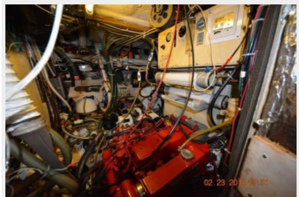
Engine room via passage way access
