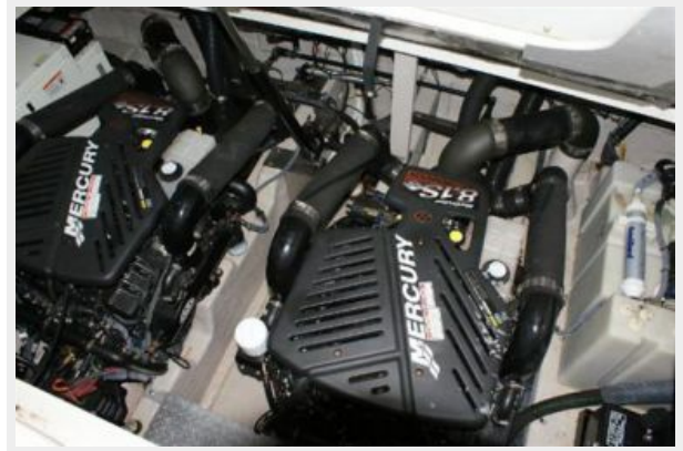
engine room detail port
