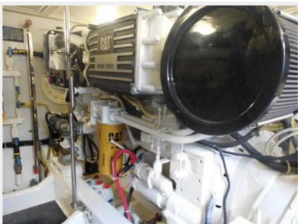
Engine Room - Cat's
