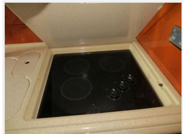
3 burner electric stove
