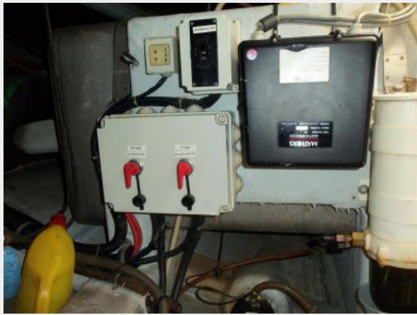
Engine Room Aft to Starboard
