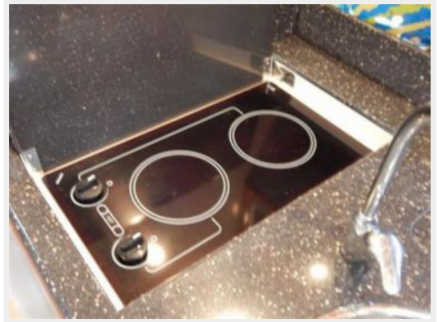
Galley Stove Top Open
