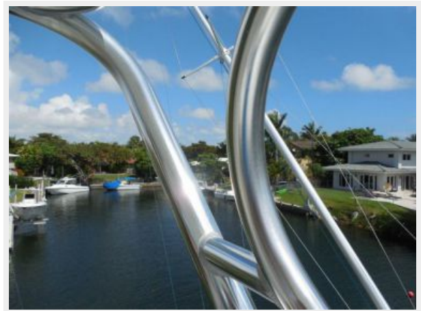
Tower Metal Condition
