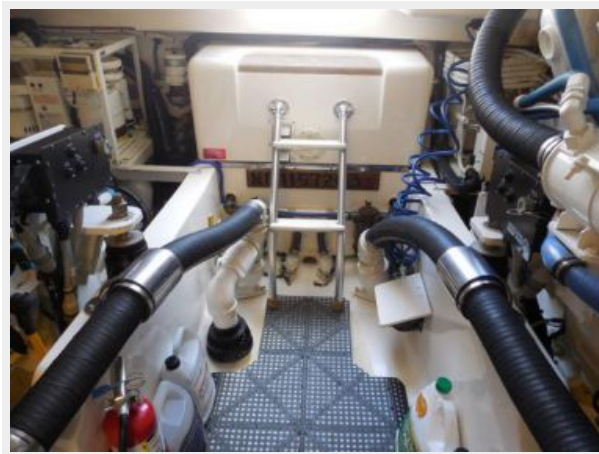
Engine Room Aft
