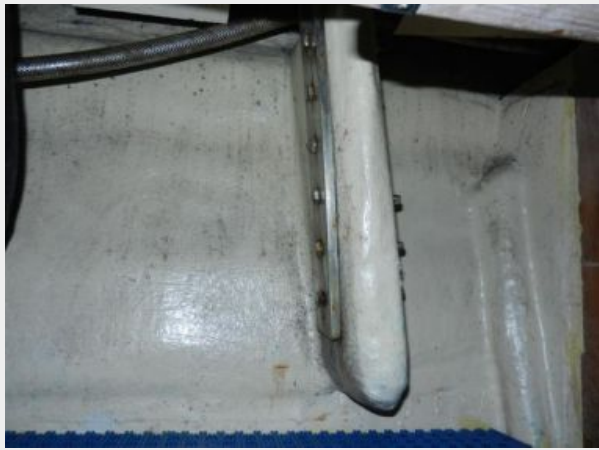
chainplate access good
