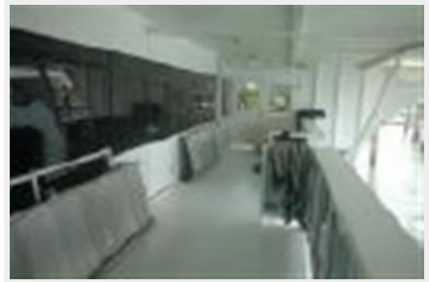
Side Deck Walkway
