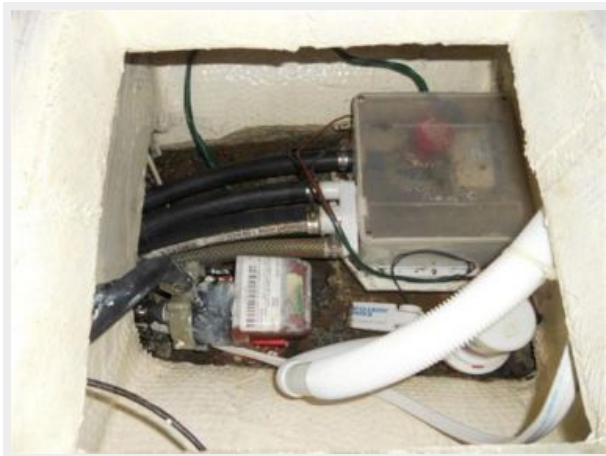
NEW SHOWER SUMP
