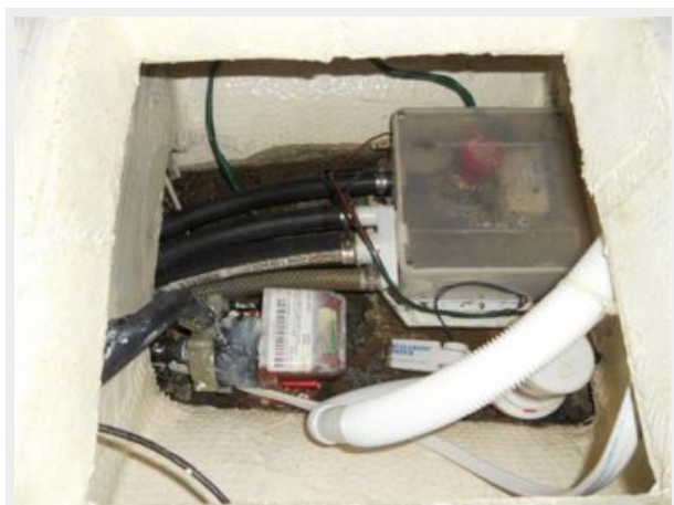
NEW SHOWER SUMP
