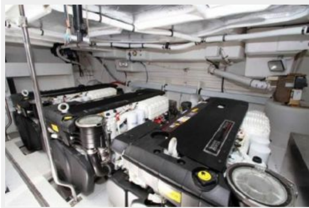
Expansive Engine Room
