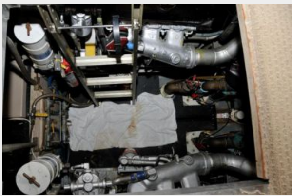
Engine Room Overview
