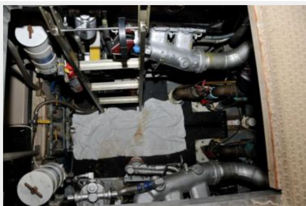
Engine Room Overview
