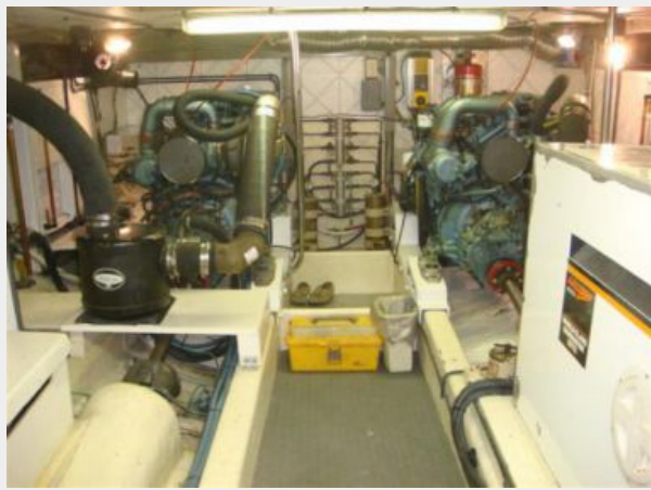
49' DeFever Engine Room Forward
