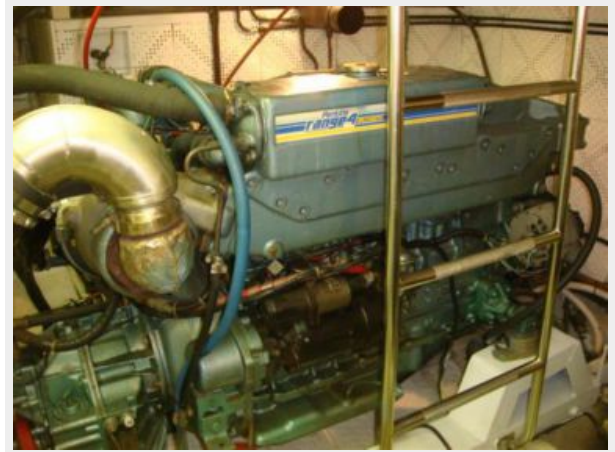
49' DeFever Port Main Engine
