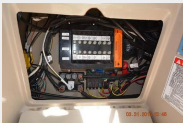
Wiring below helm
