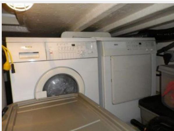
Laundry in Engine Room
