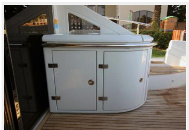
Aft Deck Electrical Panel
