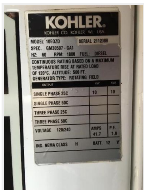
Kohler 10 kW Generator
