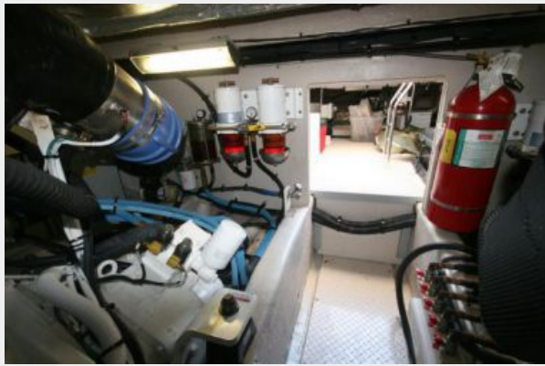
Engine Room Aft
