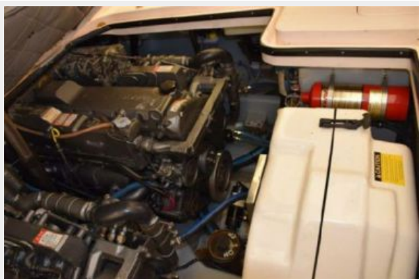
Generator in Sound Shield
