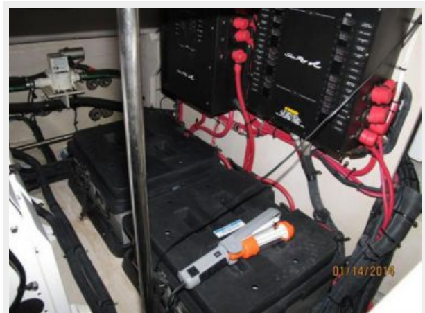
New AGM Batteries
