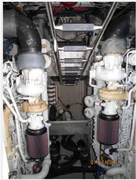
Engine Room Entry
