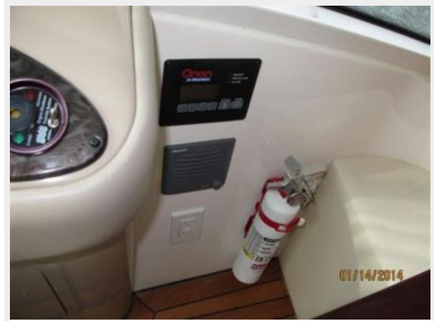
Remote Generator Panel
