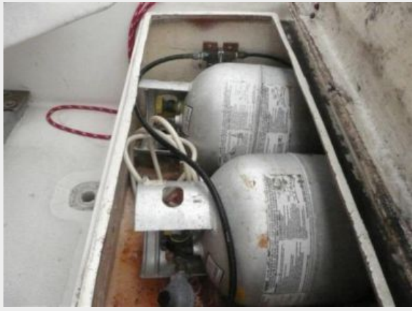
Propane Locker - Dual aluminium propane cylinders
