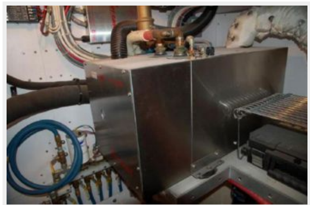
Diesel Furnace
