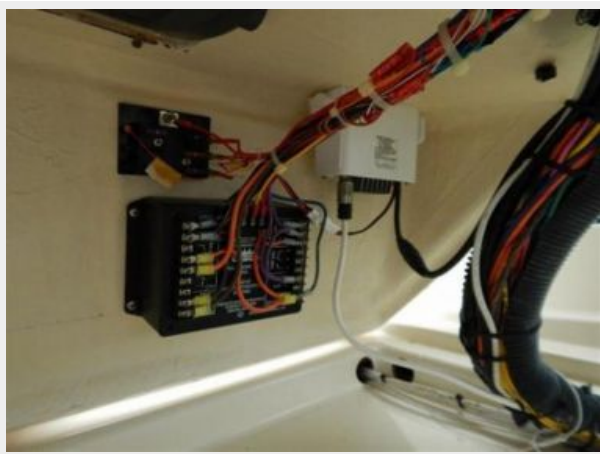
Cockpit Helm Wiring
