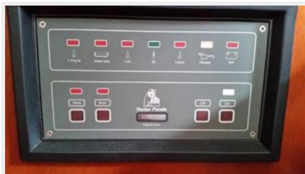
Generator Control Panel
