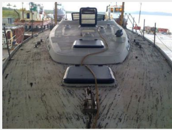
Deck "before" photo
