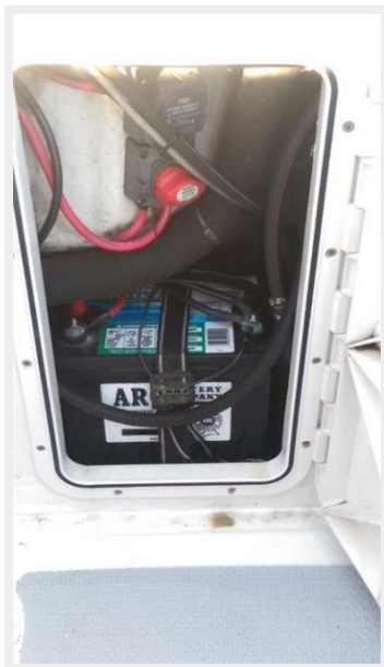
Battery & Switch - Port Side
