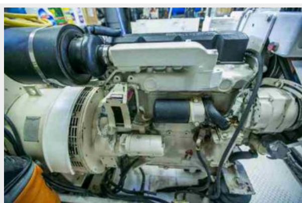
Engine room - 30kw Northern Lights GenSet
