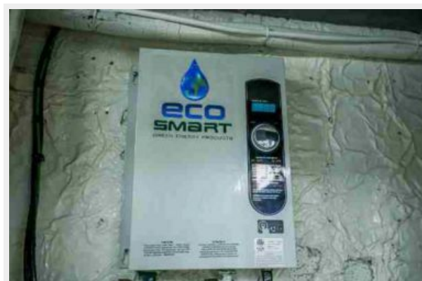
Engine room - eco smart hot water heater
