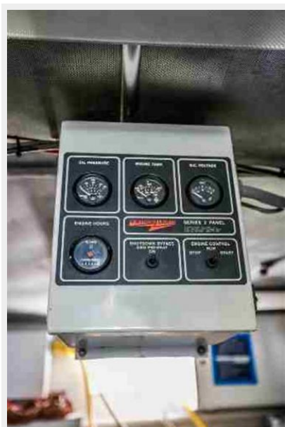
Engine Room - 30kw Northern Lights GenSet
