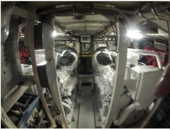
View of Engine Room
