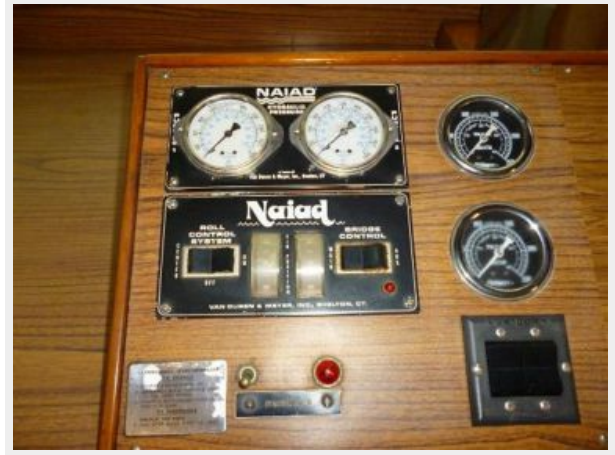
Pilothouse - Naiad Stabilizer Controls
