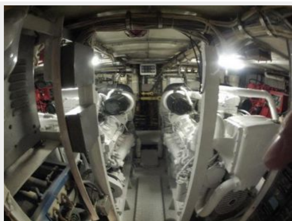
View of Engine Room
