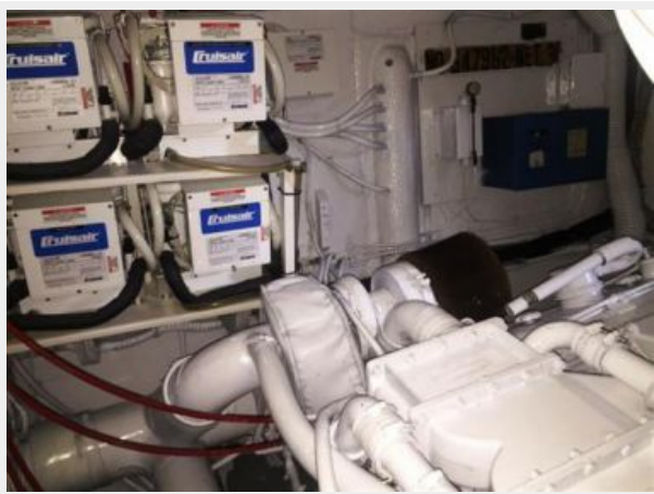
Port engine room
