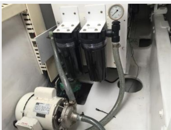
Engine Room - Watermaker Filters
