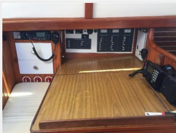
Tayana 42 - Electric Panel, VHF, On/Off Switch
