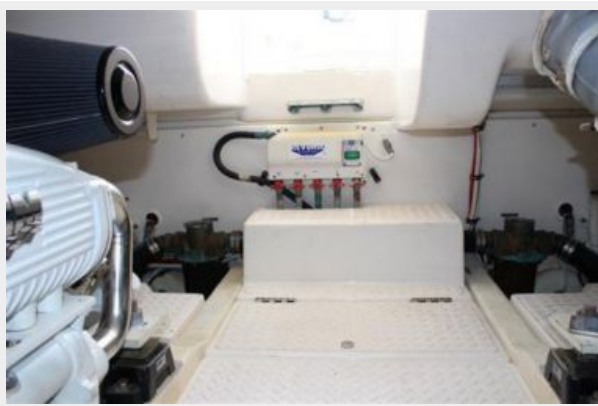
Engine room looking aft
