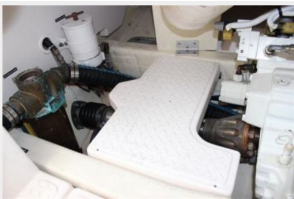
Stbd drive shaft with cover
