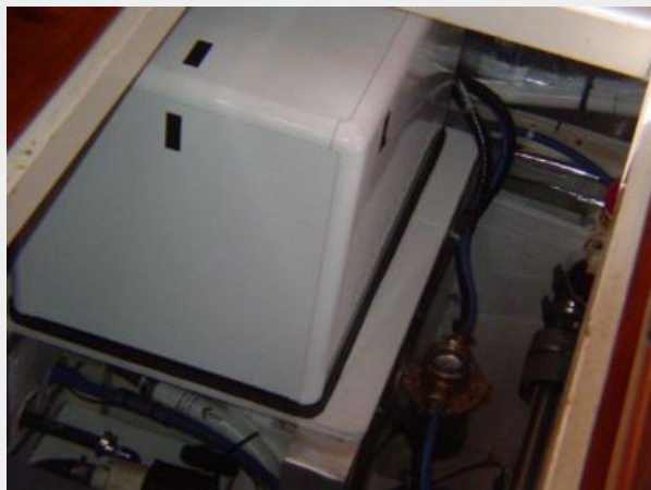
Engine Room Gen Set
