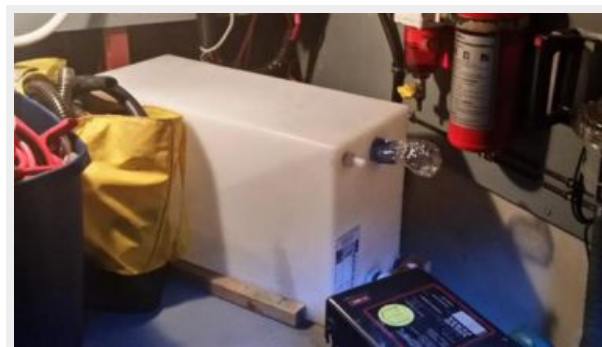
Fresh Water Engine Flush
