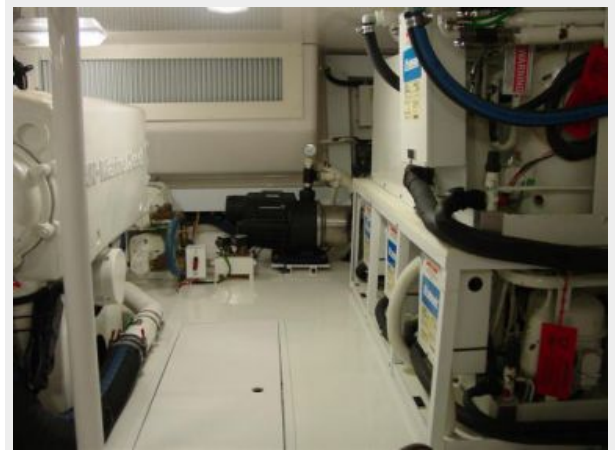
Engine & Mechanical Equipment 6
