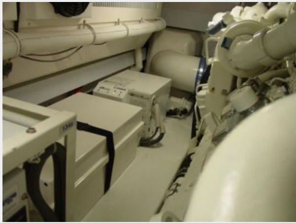
Engine & Mechanical Equipment 3
