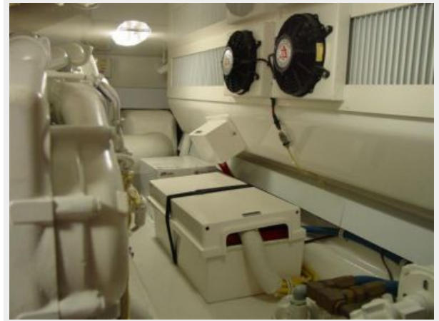
Engine & Mechanical Equipment 4
