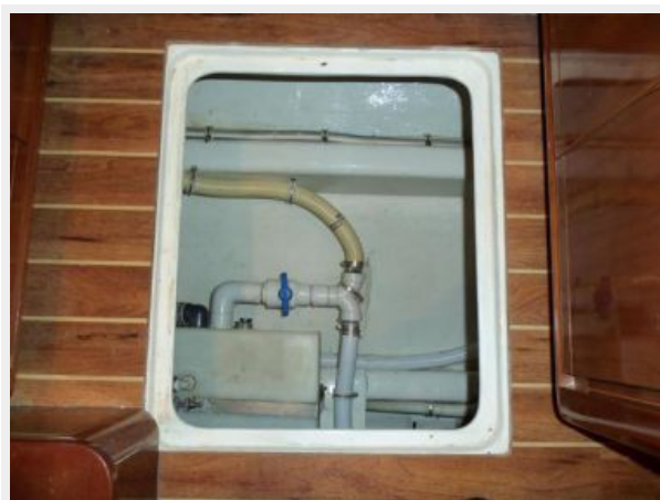
Storage Under Galley
