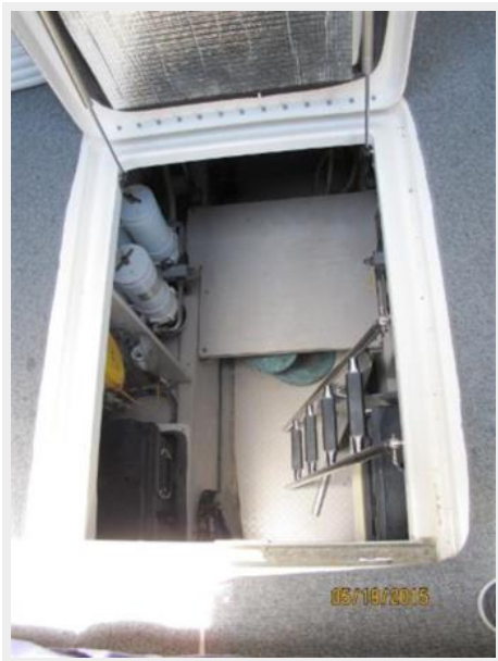
Clean Engine Room
