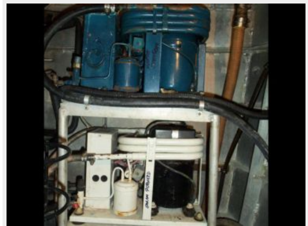
Starboard Side Lazarette
