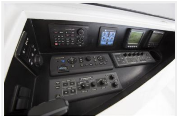
Starboard Electronics Box
