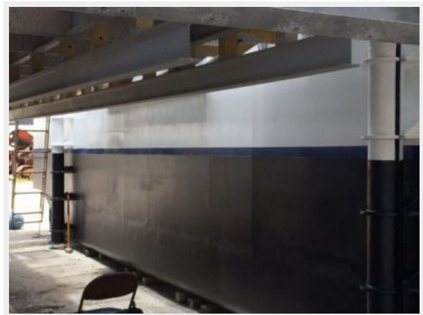
Under the lift view
