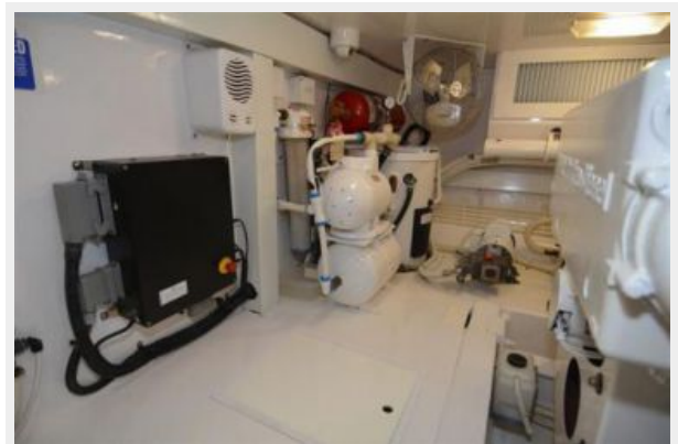
Engine Room Forward Stbd
