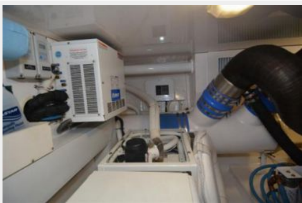
Engine Room Aft
