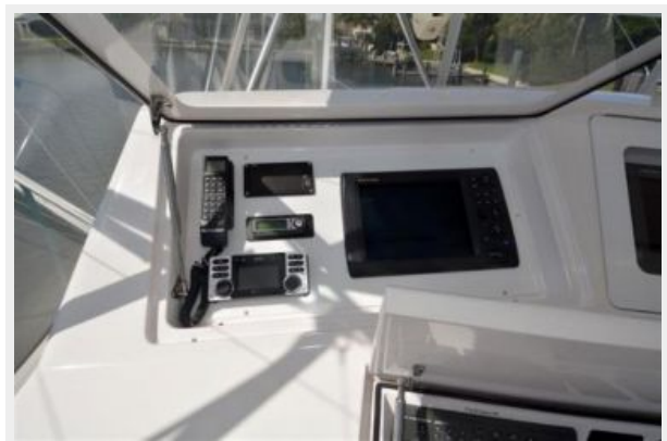
Outboard Electronics Box
