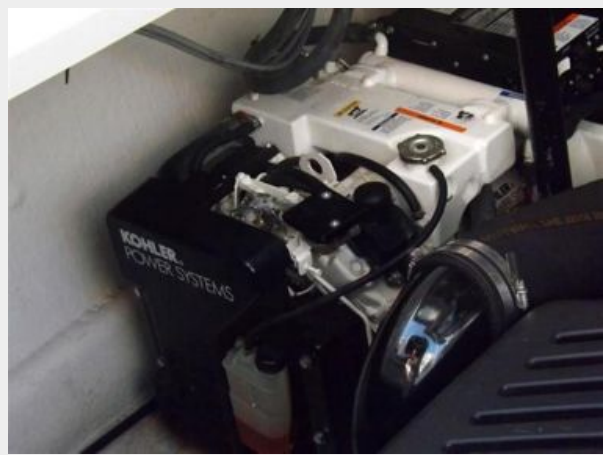
Kohler power generator 5.0kw
