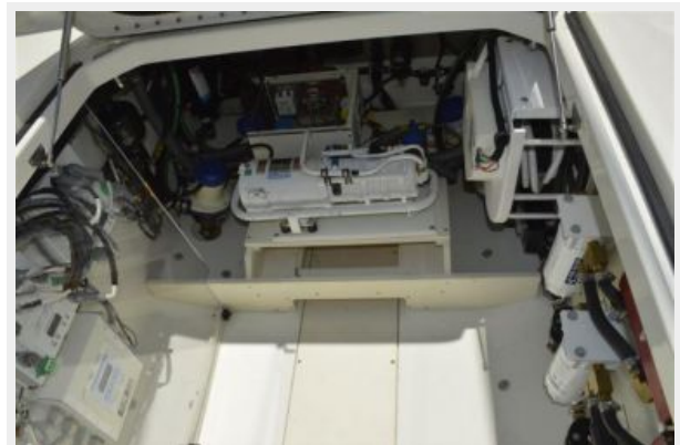
Clean Mechanical Compartment
