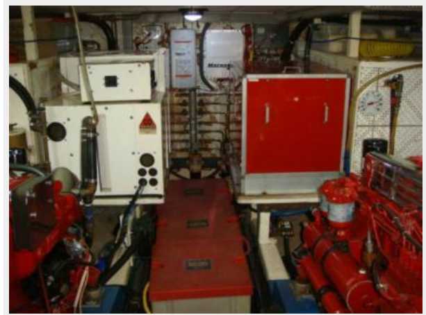
48' Defever Engine Room Aft
